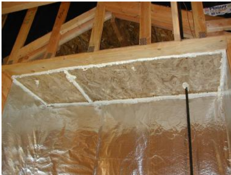
Figure 3: Draft-Stopping at Cavity for Gas Fireplace
